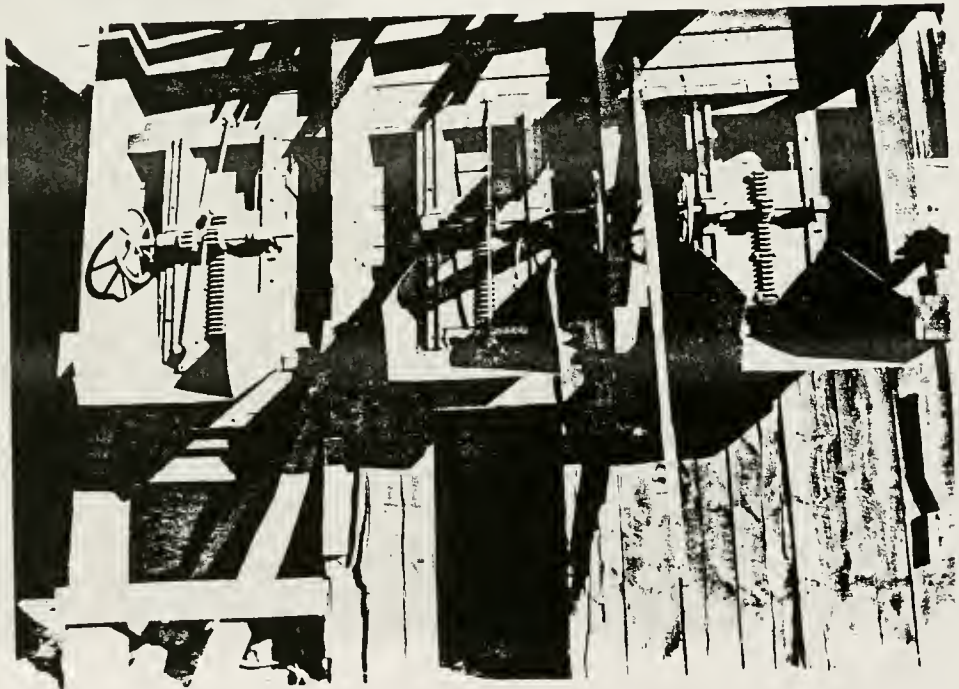
Figure 157. Arsenic plant (structure #59) showing detail of chutes on bins adjacent to McDougall roasting furnace, east view.
